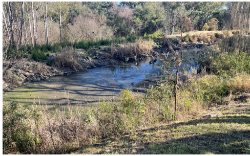
Before the repairs were done, the dam was a near-empty, stagnant mess.
