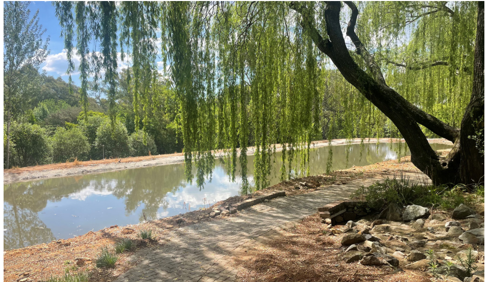
All that is left is the landscaping.
